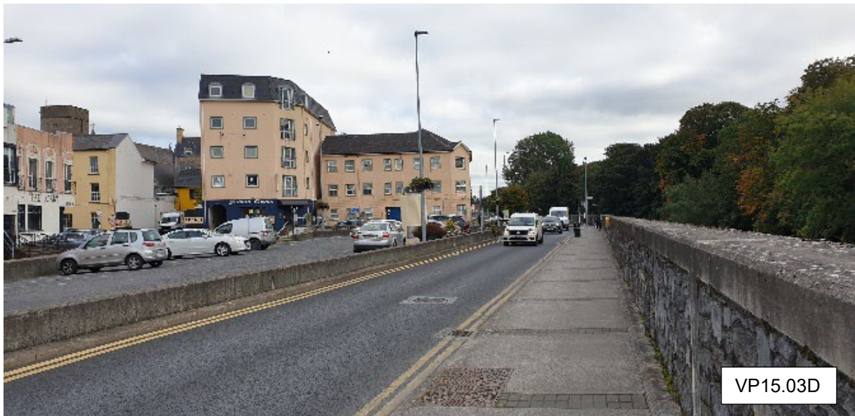
VP 15.03D Looking northeast from New Quay Road at existing carpark terminating at Sarsfield Street entry area, the proposed link for the North Bridge-01. The stone flood wall barrier is visible in the foreground on the right, and Suir Island's riverbank vegetation of mature trees.
