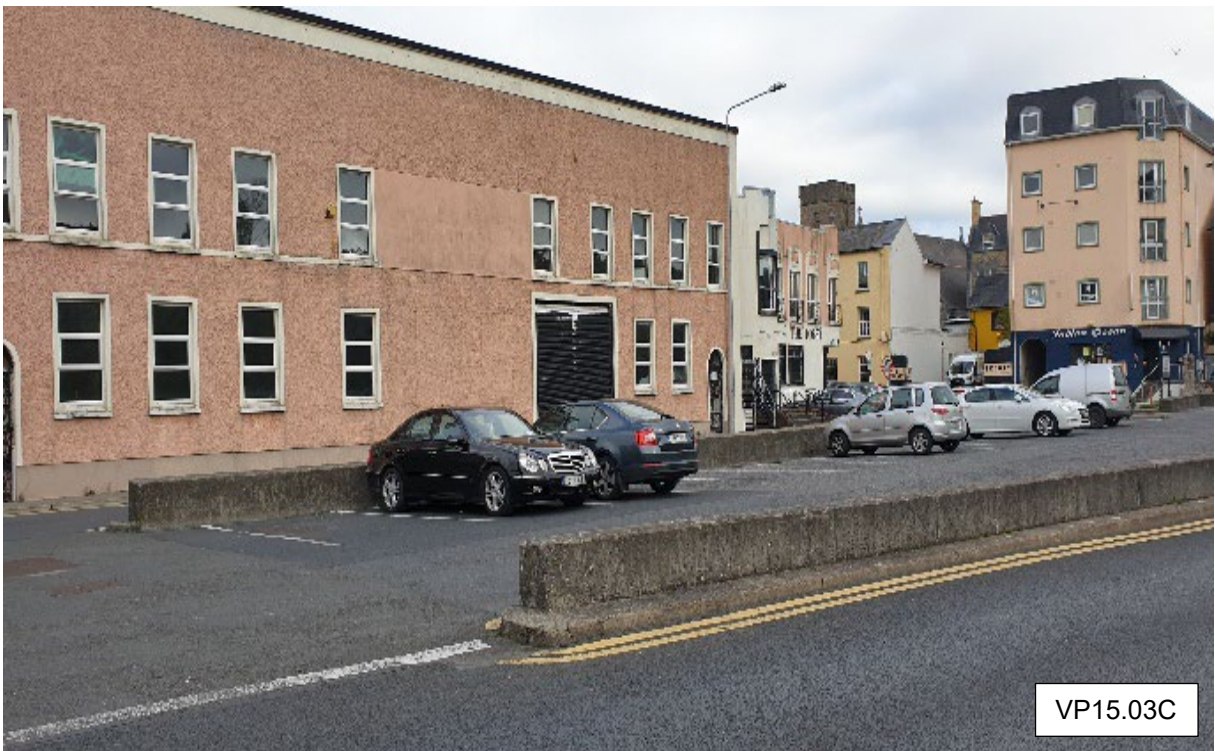
VP 15.03C Looking further northeast at the existing car park area with low concrete walls.
