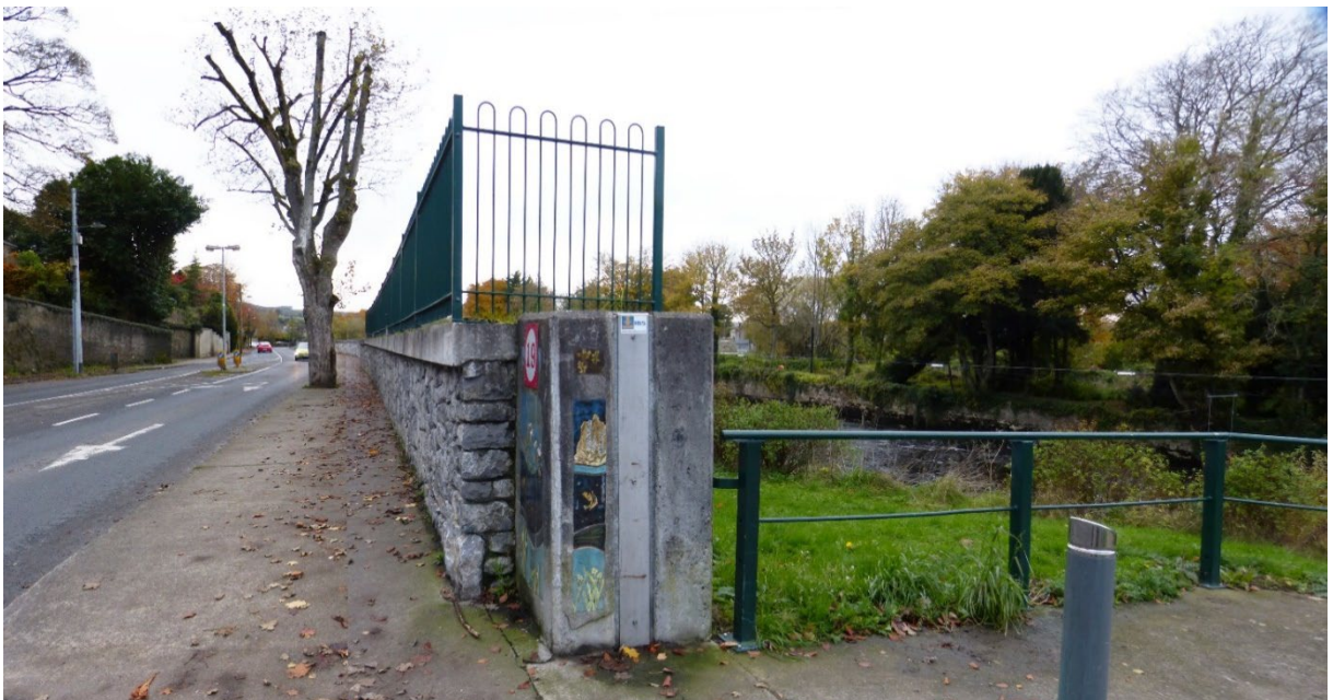
Image 15.4_08A From Denis Burke Park entrance looking West (Existing view).
